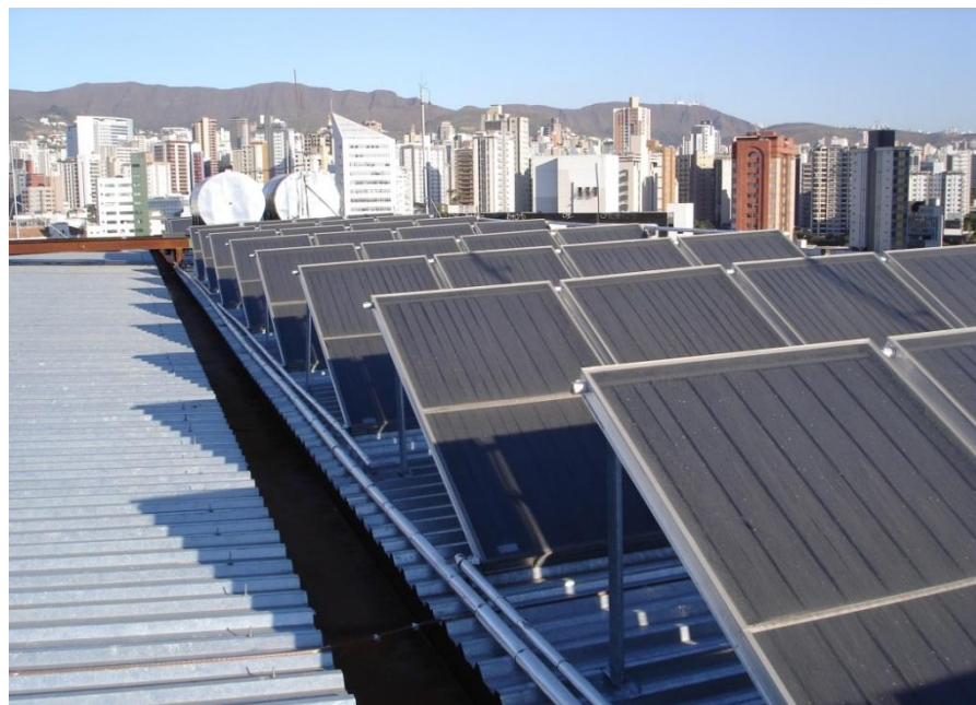
Hospital João XXIII
